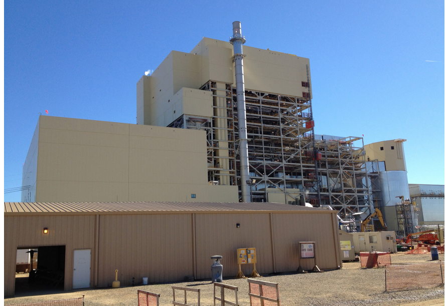
Virginia City Power Plant > St. Paul, VA
