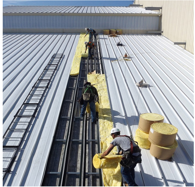
Southwest Airlines Re-Roof > Orlando, FL
